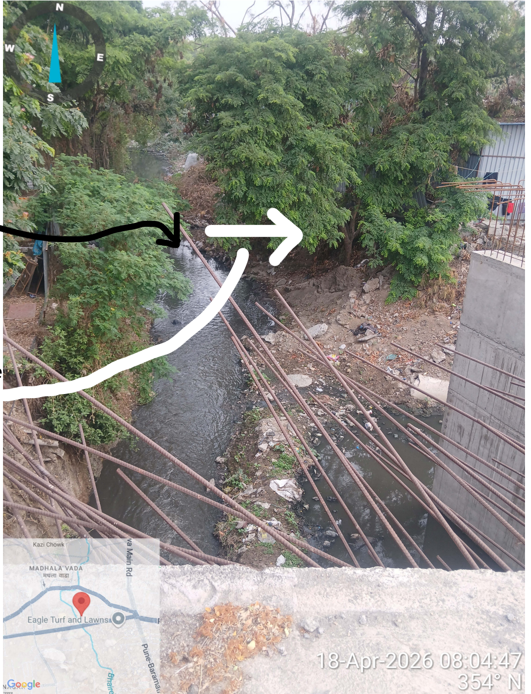
Figure 3: Photograph showing illegal obstruction of Bhairoba Nullah and diversion of its water course at an angle of 90 degrees
